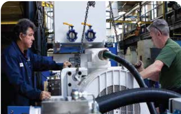
PRESSURE SYSTEM REPAIRS
